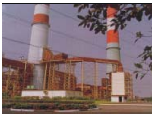
FGD Plant at TPC Fig – 4
