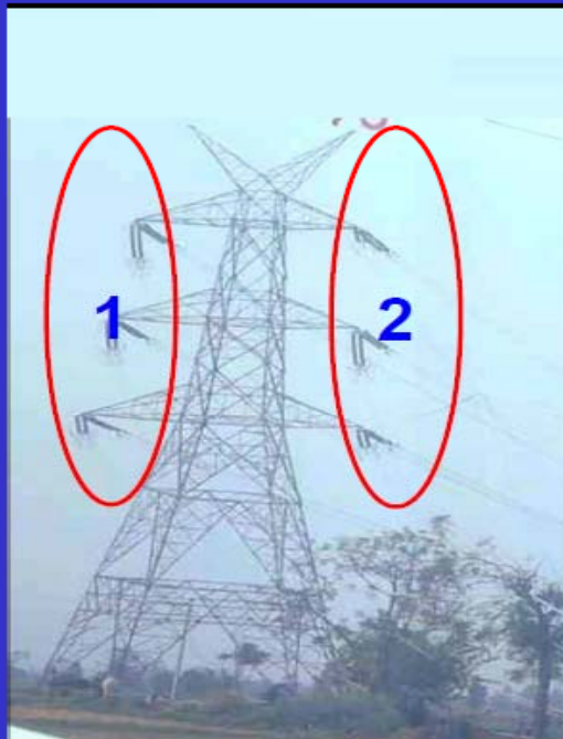
DOUBLE CIRCUIT TOWER
