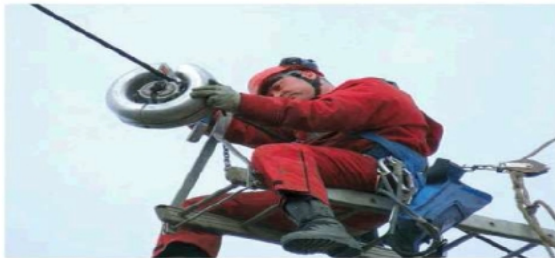
Fig 2.installation of power donuts
