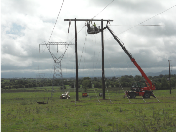
Figure 6. Temporary stringing structure
