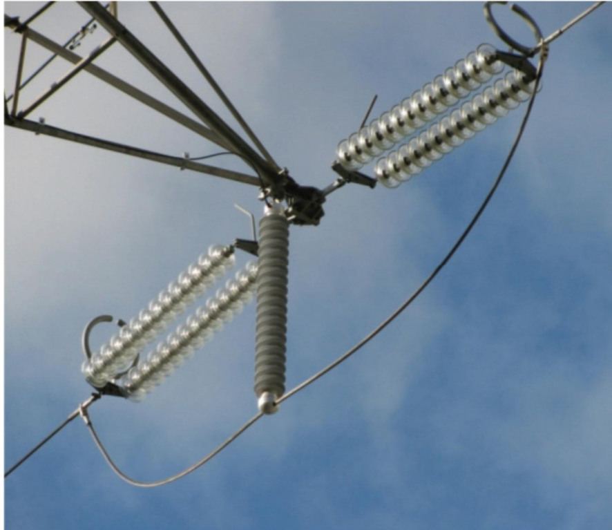
Figure 21. FibreSensing system installed [71].
