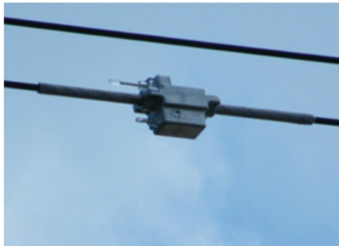
Figure 14. Ampacimon sensor installed on the line (with armour rods). [42]
