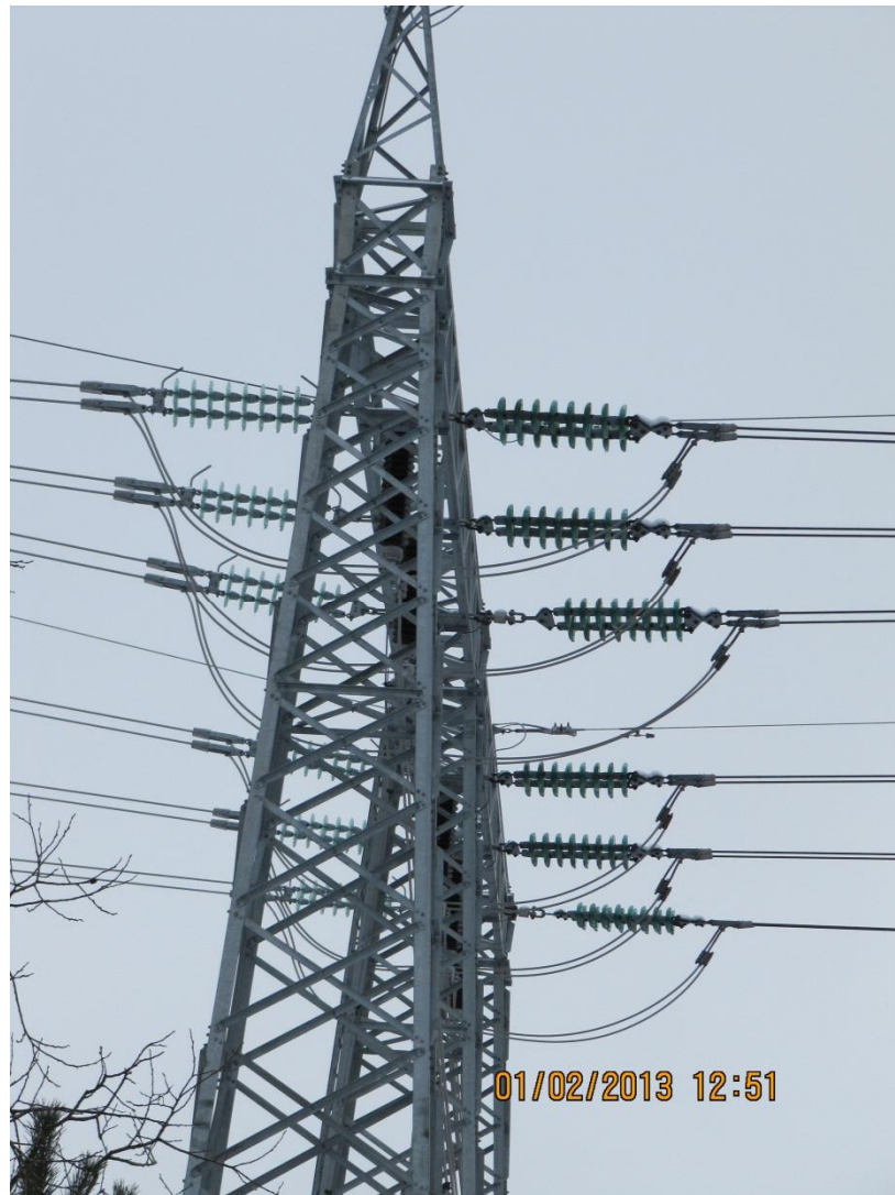
Figure 27. CAT-1 load cells installed between the tower structure and the insulator strings on the further-most phases of the two circuits. Simolantie, Lappeenranta.[31]
