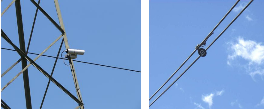
Figure 13. Sagometer camera mounted on a tower (left) and the target mounted on the power line (right). [36], [37]
